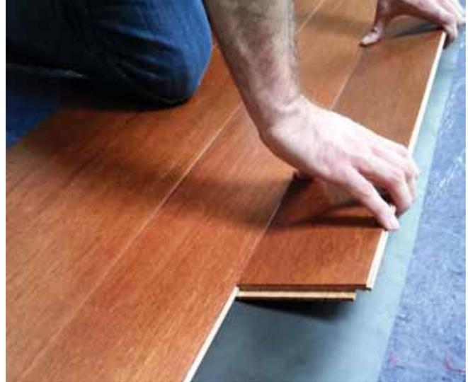
After temporarily placing a section of 6” by 48” felt paper under the leading edge between the floor and underlayment, simply slide the paper along the leading edge during board assembly. This prevents the locking joints from pinching the underlayment. Pull the paper along the leading edge until a row is completed.
