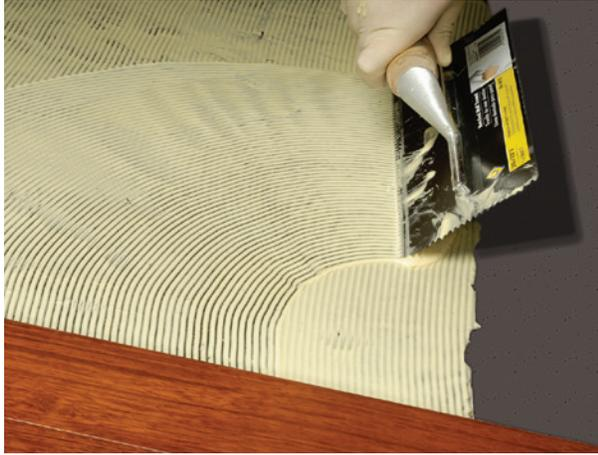
the moisture content of substrate exceeds or is within the flooring manufacturer's recommendations, to address current or possible future subfloor moisture, sound, and cracks (up to 1/8"), apply Bostik's BEST® as directed.
